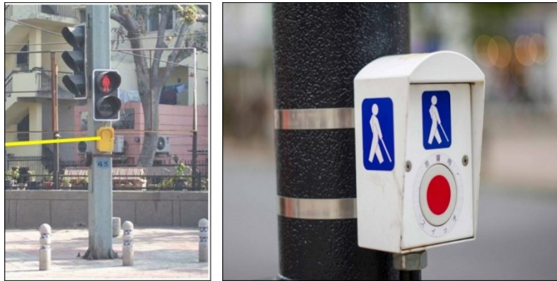
Photo- 3.12 Traffic signal, bus rapid transit, Delhi (left) and audio signal (right)
