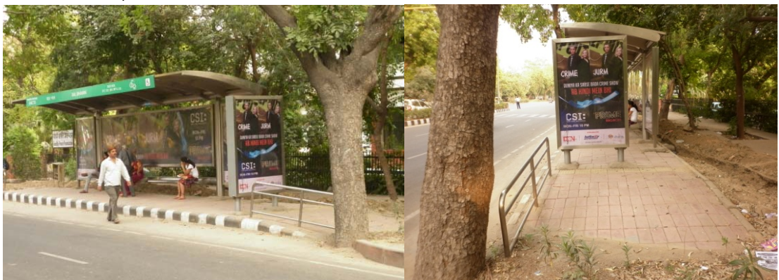
Photo- 4.1 Handrails are not accessible due to incorrect placement
