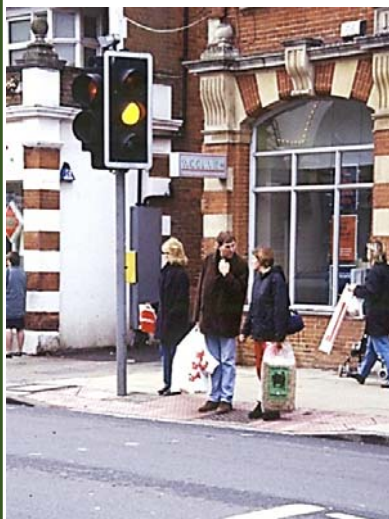
Pedestrian Pelican Signals for light-controlled crossing and tactile paving
