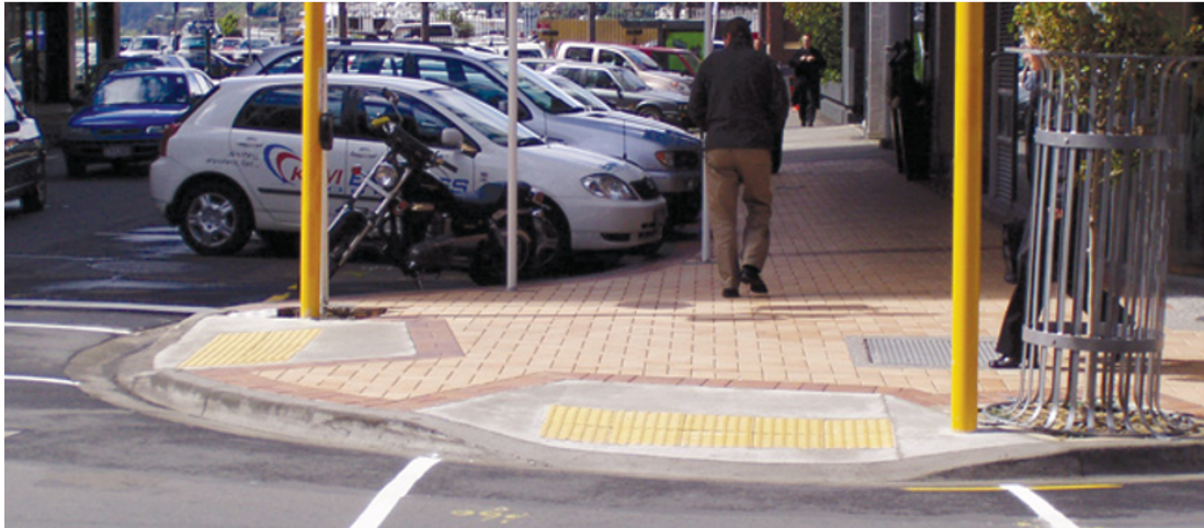
Photo 3.1 -Kerb ramps with tactile warning pavers at transition points
