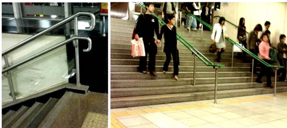
Photo 3.4 Rounded handrails ends
