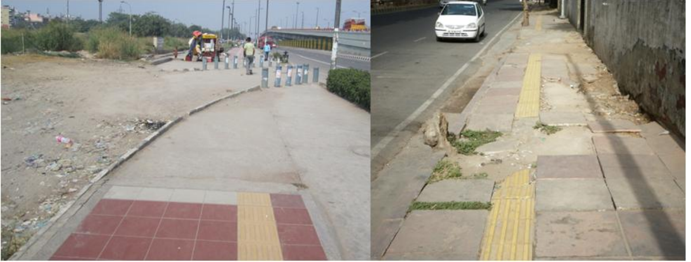
Photo 2.4 -Incomplete tactile path and un-maintained footpaths.
