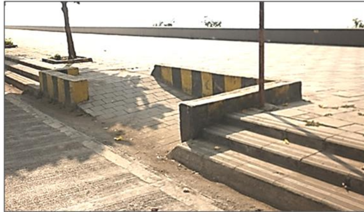
Photo 2.3 Access audit implementaion, Mumbai
