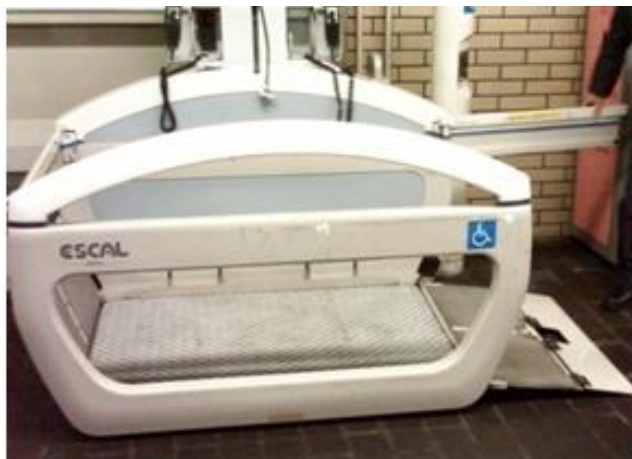
Photo 3.2 Hydraulic stair lift
