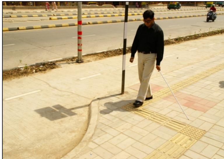
Photo 3.5 Tactile pavers in open areas
